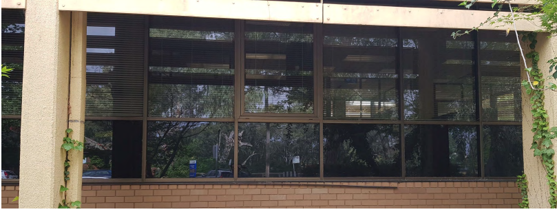
G Existing Aluminium Framed Windows & Colourback Glass Spandrels
