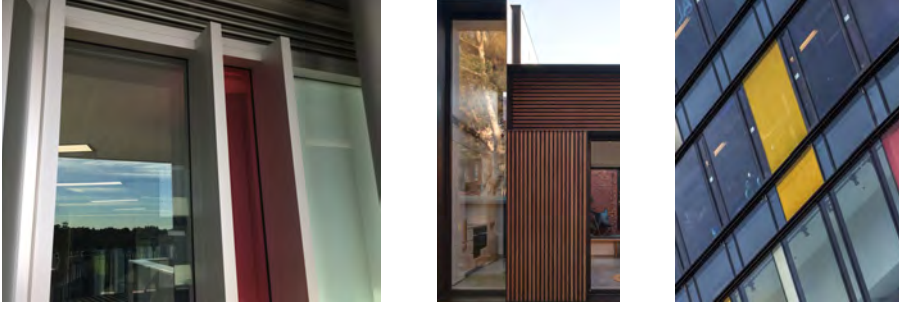
H New Aluminium Framed Windows & Colourback Glass Panels
